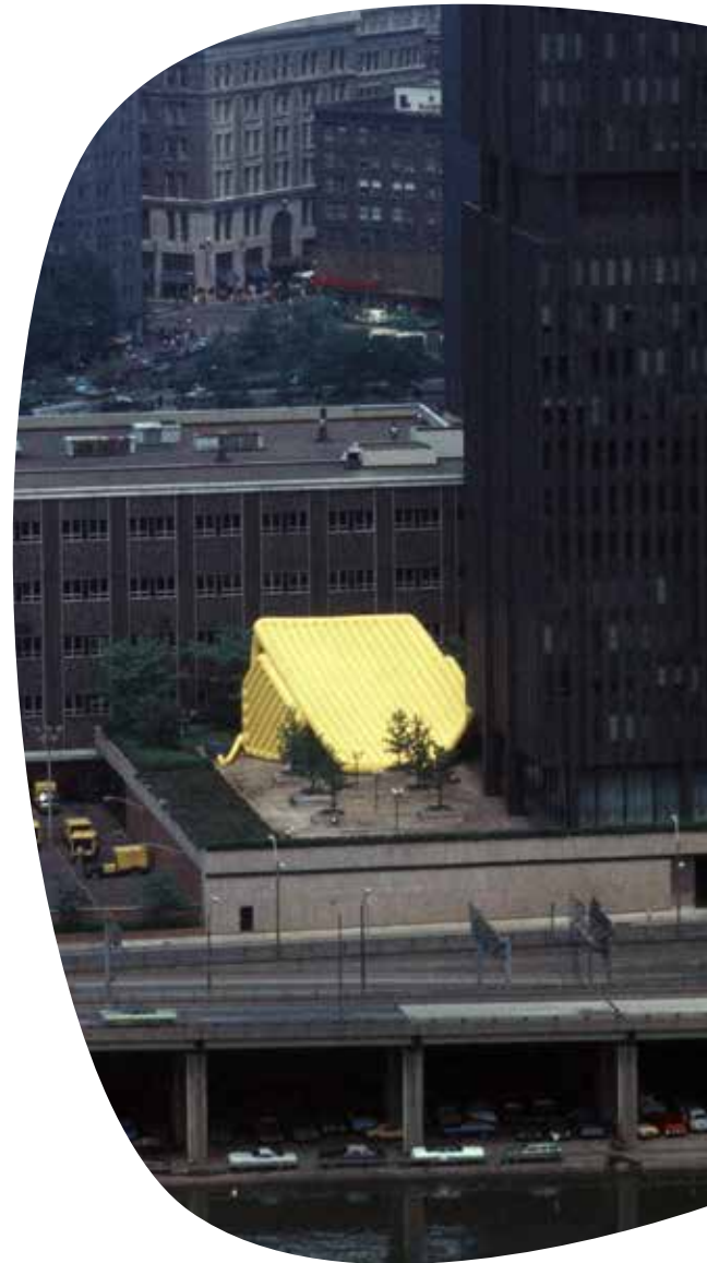
Fabricated in collaboration with architecture students at University of Wisconsin-Milwaukee, the Three Rivers double-layered pneumatic membrane performed as a seasonal event-space on Westinghouse Plaza for ten years.
