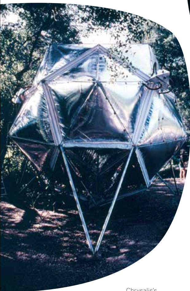
Chrysalis's Dodecahedron (1970)—a lightweight metal frame with infill panels of mirrored Mylar—commissioned by Jantzen to photograph their new swimsuit collection. A network of pneumatic tubes, visible on the far right and left sides of the construction, regulates the inflation of each panel, anticipating the logic of what is now known as ETFE (ethylene tetrafluoroethylene) cushion systems.
