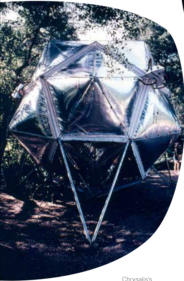
Chrysalis's Dodecahedron (1970)—a lightweight metal frame with infill panels of mirrored Mylar—commissioned by Jantzen to photograph their new swimsuit collection. A network of pneumatic tubes, visible on the far right and left sides of the construction, regulates the inflation of each panel, anticipating the logic of what is now known as ETFE (ethylene tetrafluoroethylene) cushion systems.
